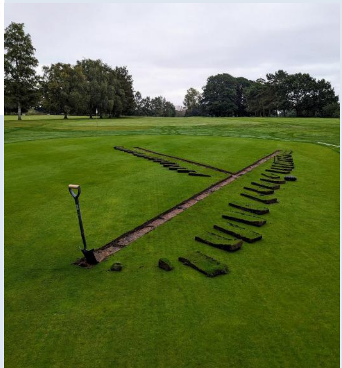
The new drain installed on the 9 th green has really been put to the test this month. Although it has not totally cured the problem, there is an improvement and water is being removed from the green.
